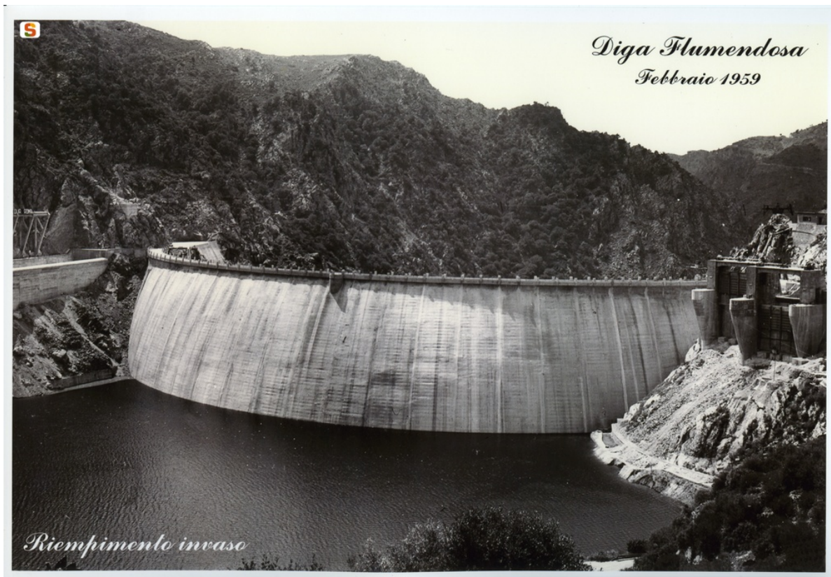
Figure A.2: Picture of Flumendosa Dam (Sardinia, 1959)
